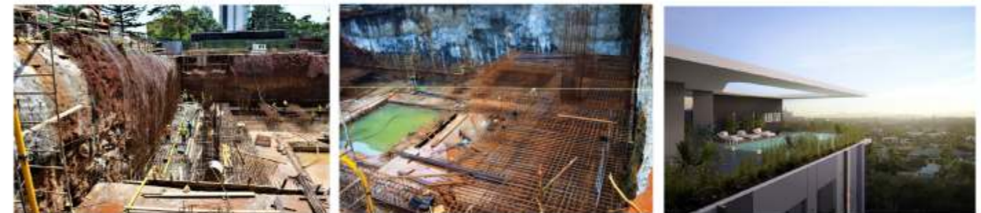
Habitat Apartments under construction
