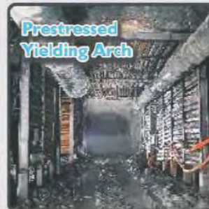
Yielding Arch Sets This system enables the support set to be an active unit at 7.5 ton/meter 2 suitable for portals and unstable areas where access to the workings are required.
