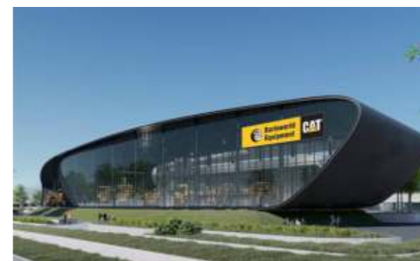
Rear view of the showroom.
