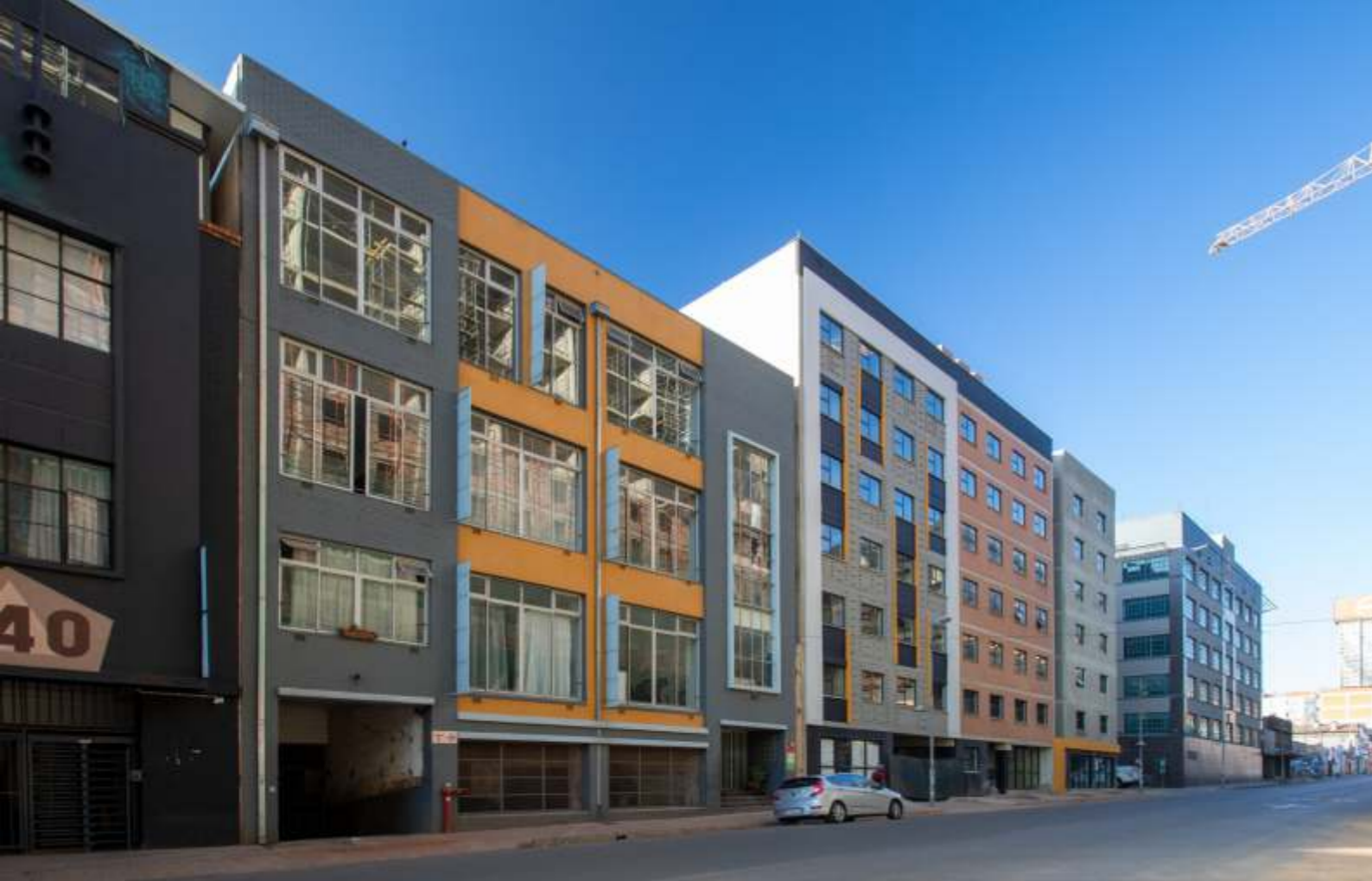
Divercity - external view of the residential rental apartments
