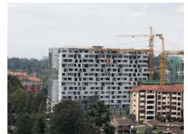
Purple haze apartments at almost completion stage.
