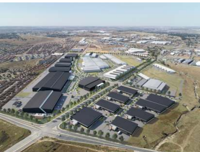
Aerial view of Sterling Industrial Park development by Growthpoint
