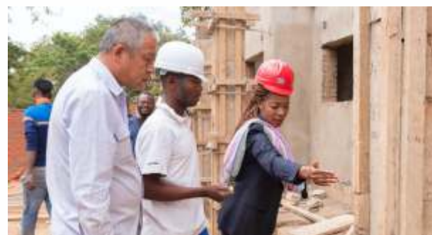
Mdoko supervising construction works.
