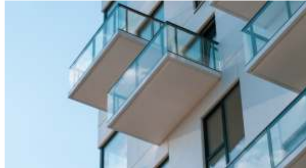
An apartment unit with balcony.
