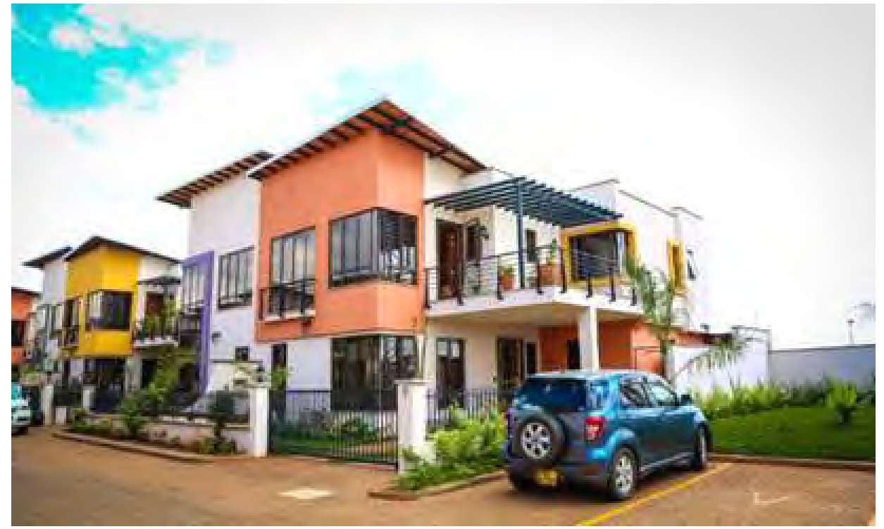
Phase 1 of the townhouses consisting 66 units are currently fully sold and occupied.
