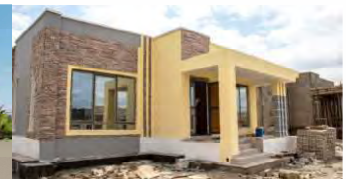
Almost complete unit
