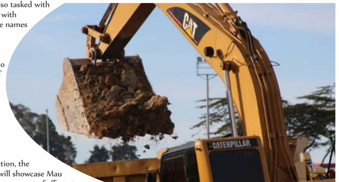
Ongoing road construction project.
