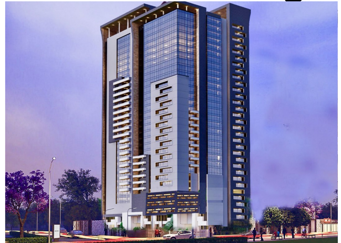
Construction of the much anticipated Rama Towers, an ultramodern mixed use development in Kilimani, Nairobi, is set to begin shortly.
