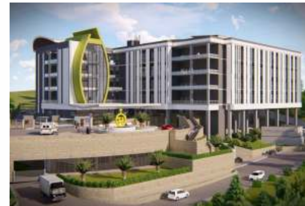
Tenwek Hospital in Bomet will soon have a new Cardiothoracic and Emergency Centre.
