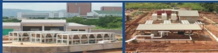
COURT OF APPEAL HQ AND ABUJA DIVISION, ABUJA
