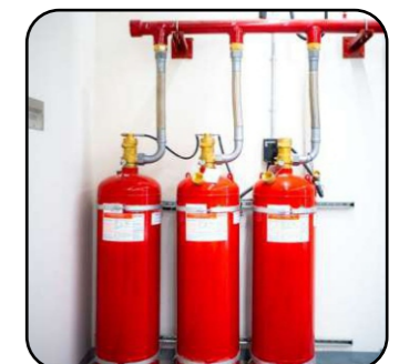
Automatic Fire Suppression Systems
