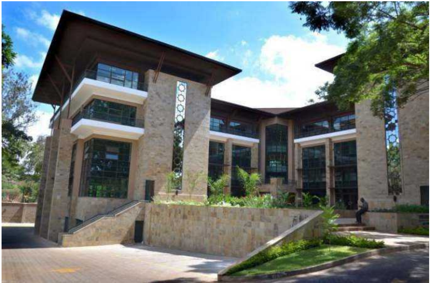
Office Development On General Mathenge Drive, Nairobi
